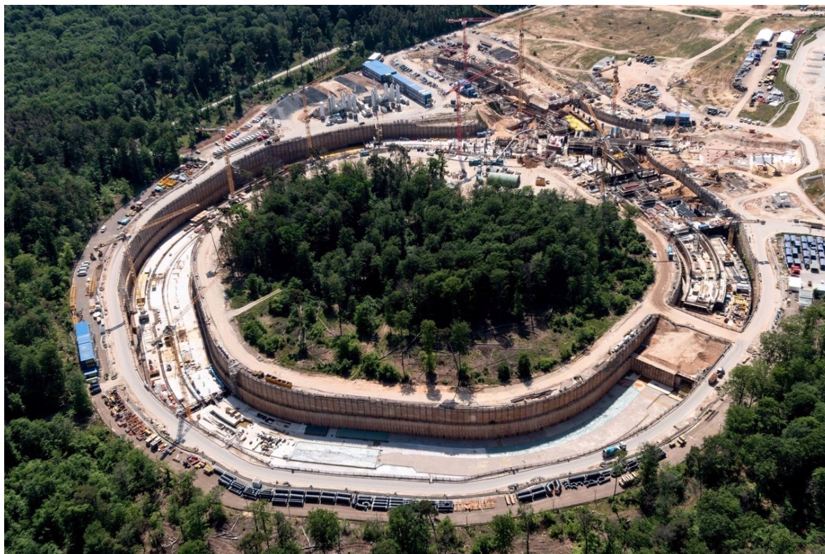
Figure 4. The FAIR construction site in spring 2020. The picture shows the progress in civil construction for the SIS 100 tunnel, the 'transfer building', where the beam delivery from the existing and upgraded GSI accelerator chain into the SIS 100 and also the delivery from the SIS 100 to the various FAIR experimental sites will occur, and the cave which will hold the CBM experiment. Now, in winter 2022/3 the SIS100 tunnel is closed and the civil construction on the south campus (upper right part in the figure) has nearly been completed. The first science experiments are scheduled to start in 2027. Credit: GSI.
